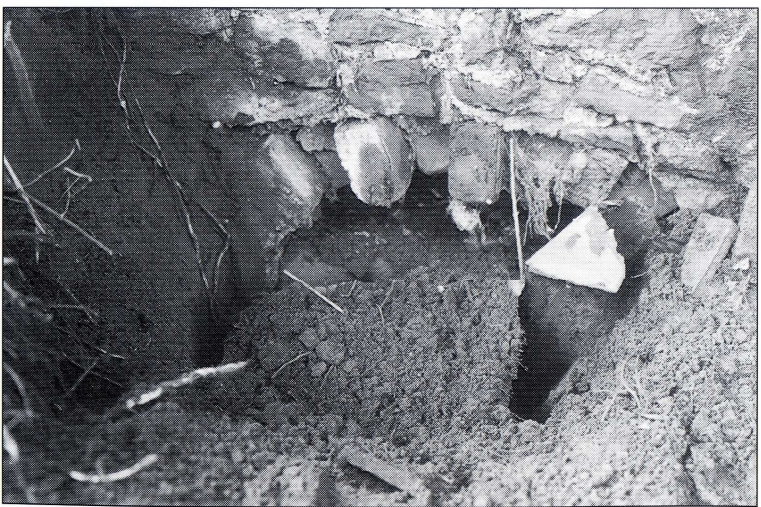
The remains of the arch revealed behind the corrugated iron sheet on the side wall of Peter Gellatly's privy near Shere. (Roy Drysdale)
