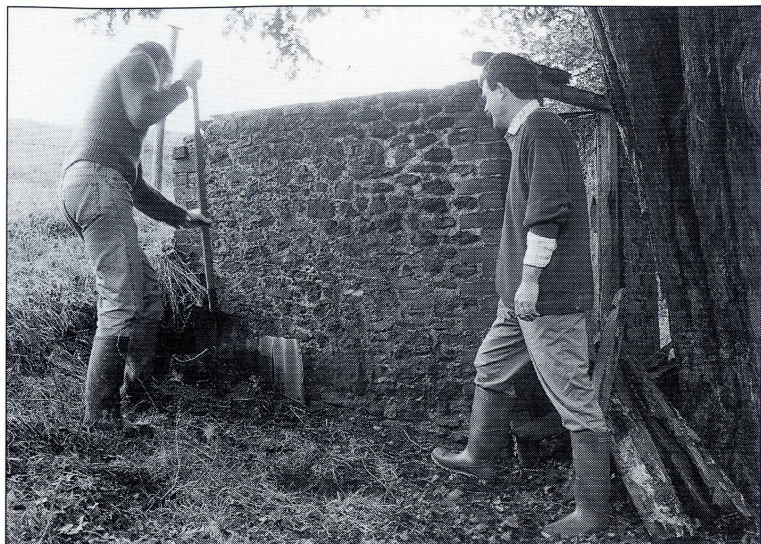
The author looks on as Peter Gellatly digs into the bank in the hope of finding the arch of a dry privy behind the sheet of corrugated iron. (Roy Drysdale)
