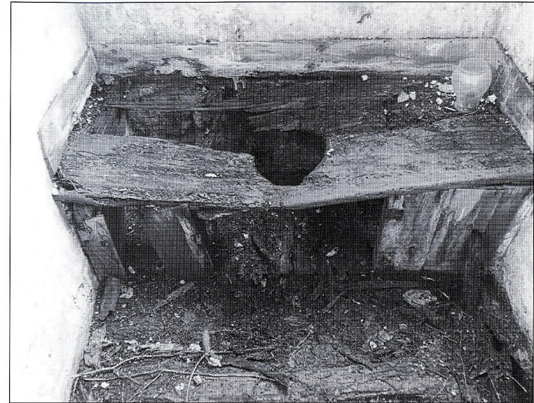
Inside Peter Gellatly's privy near Shere I found the glass jar for the candle still in position in the corner of the seat. (Roy Drysdale)
